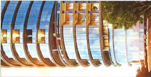
SEGMENTED CURVED GLASS FACADE
