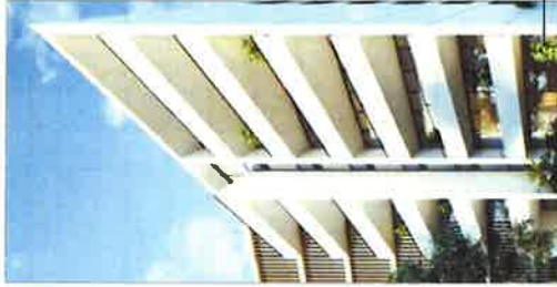
BALCONY SPANDREL PANELS
